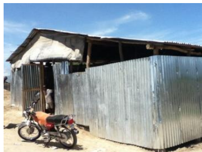
Building used for "Restoration Center", Barahona, Dominican Republic
